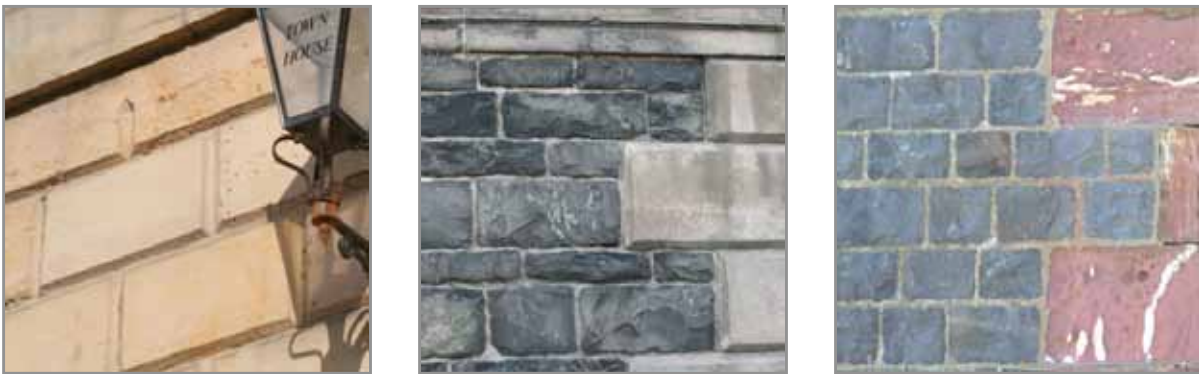
Moray Yellow Sandstone (L) local Whinstone (centre) and Whinstone combined with Turriff Red Sandstone (R).
