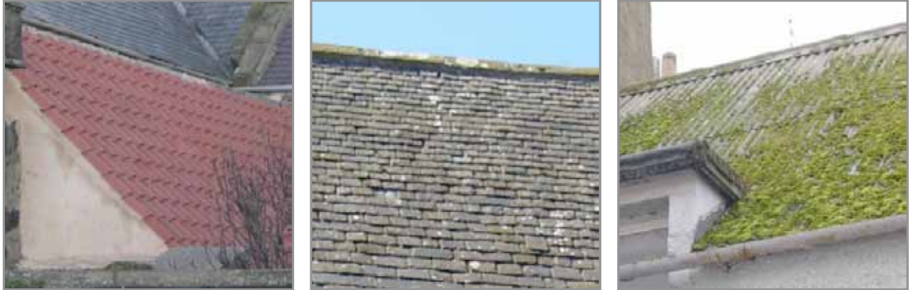
New clay pantiles (L); traditional Scots graded slate roof (centre); aging asbestos roof (R) which can be seen on a number of buildings in Banff
