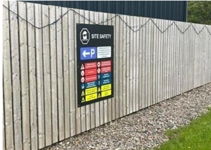
Figure 1 – Example of signage on display in a prominent position to advise of site rules.
