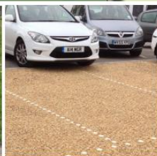
Geogrid Surfacing to Parking Bays
