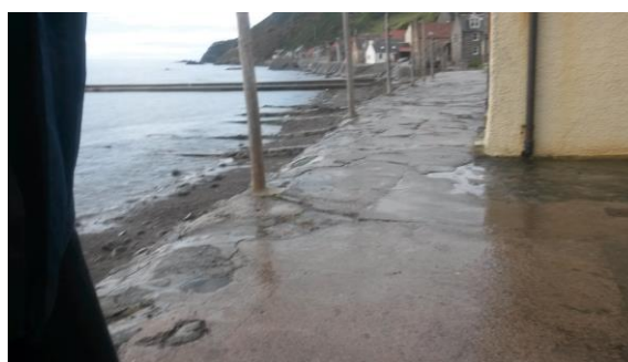
Fig 22 – Bankhead: Posts, Stone and Concrete
