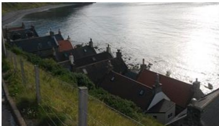
Fig 15 – Image of Roofs with Various Finishes
