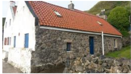
Fig 18 – Rebuilt on earlier footings
