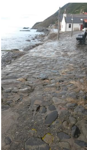
Fig 27 – Beach Stone & Concrete Hardstanding
