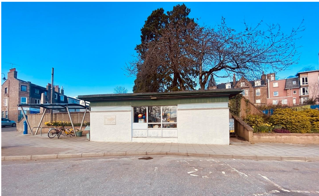
Image 1 – Front elevation of property, March 2024
