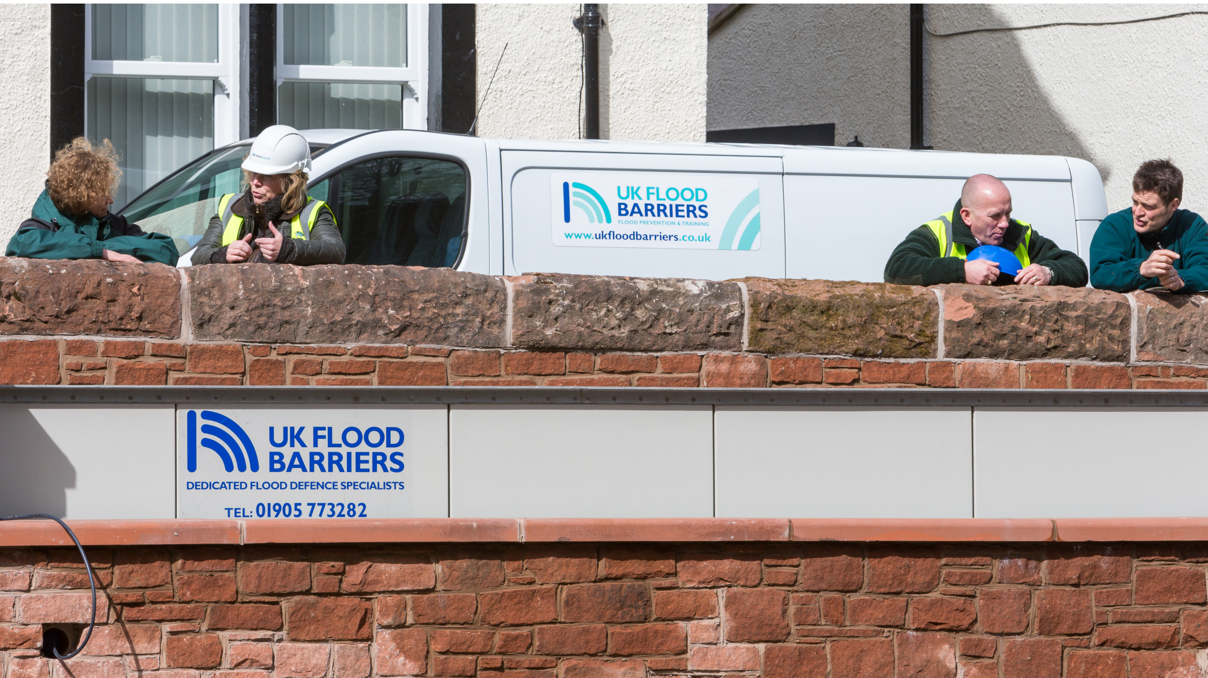
[below] Final testing of the scheme, with the barriers partly deployed. Note the use of local red sandstone for the coping and cladding of the upgraded wall.
