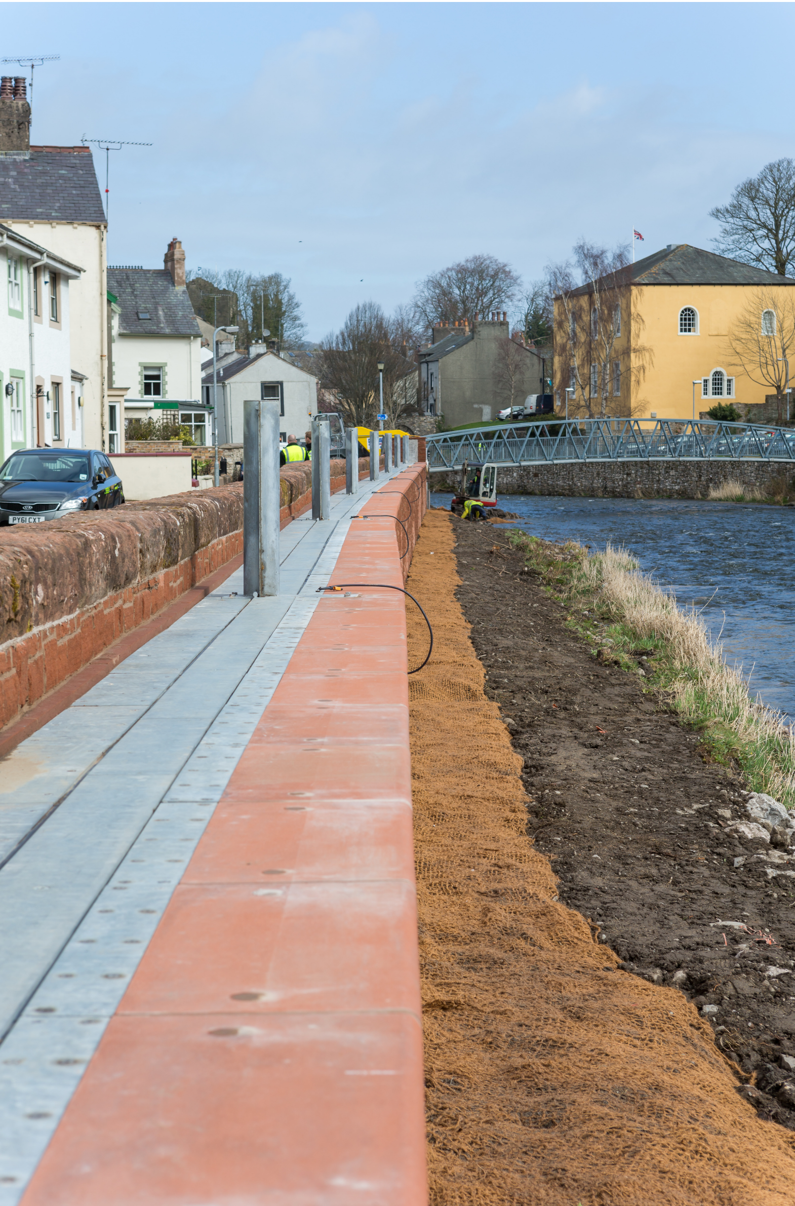
[below] Testing of the barrier, with coir matting along the base of the wall to encourage vegetation.
