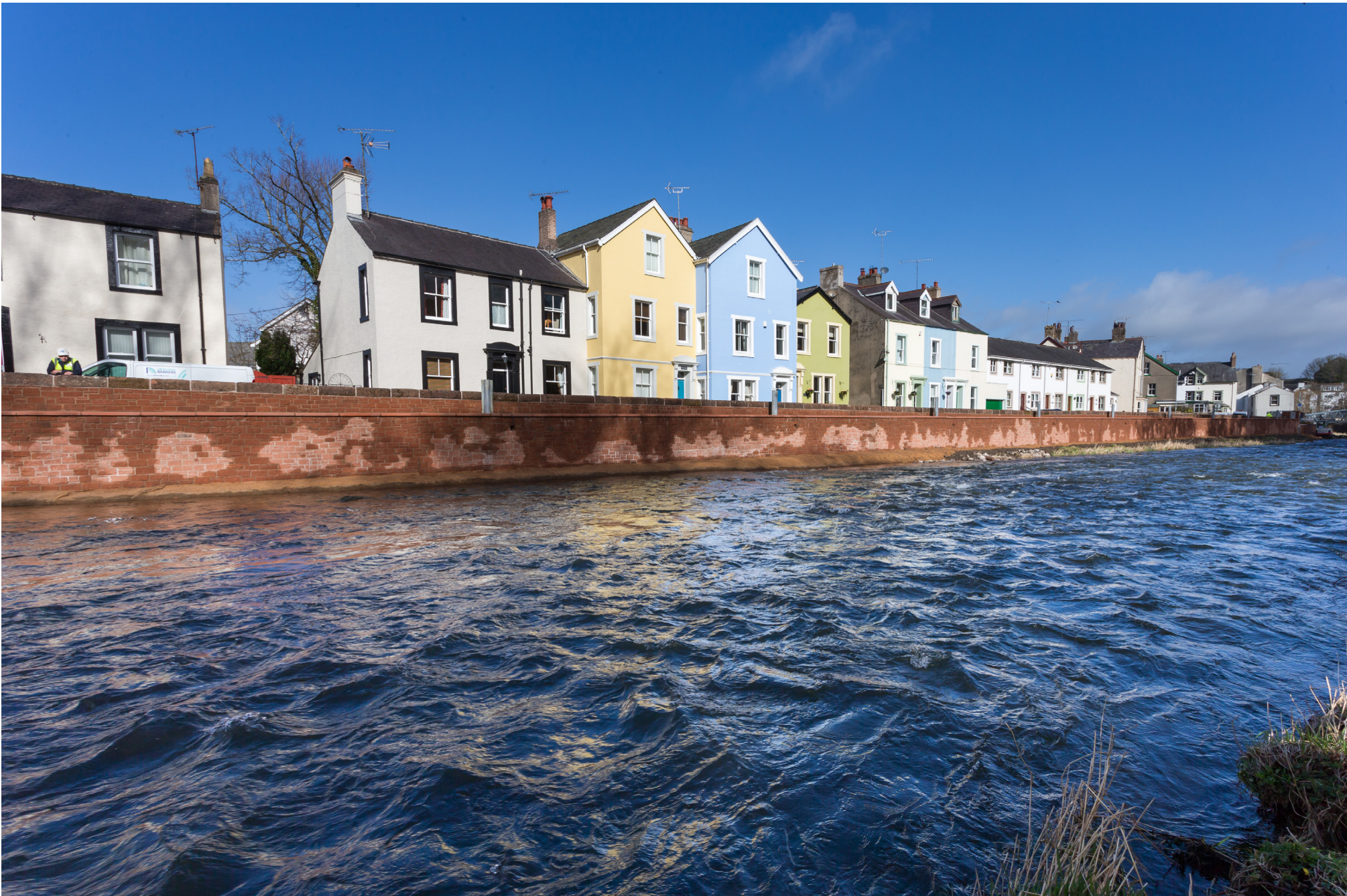
[above] The Cockermouth scheme fully deployed, with an additional 1m of protection above the existing wall. [below] When in the 'resting' position, the barriers are protected within the wall and do not impact on the attractive riverside views.
